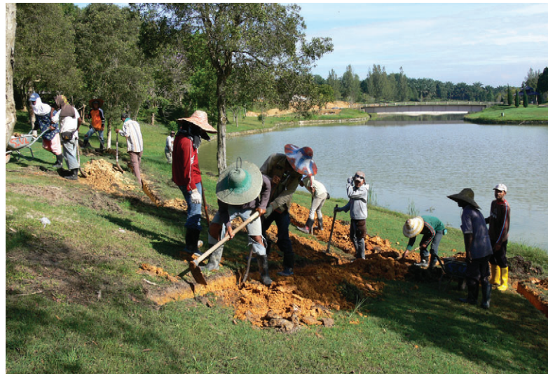
Digging drains, Malaysia
