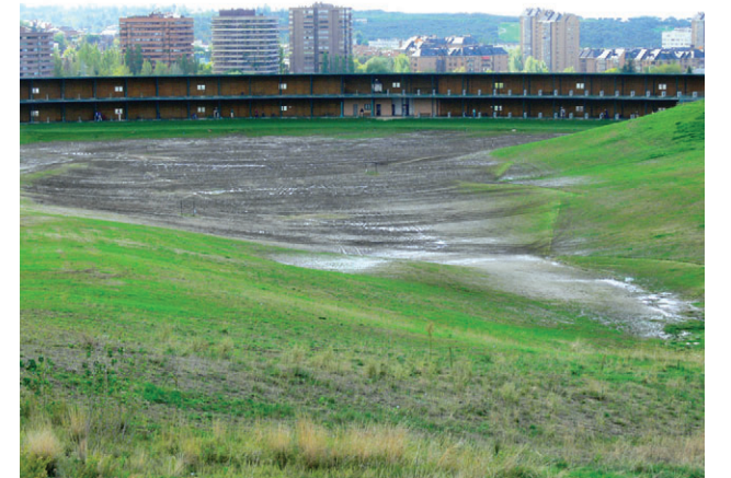
Poor drainage reduces potential revenue
